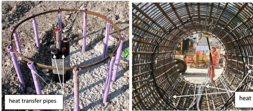
Figure 1: Heat transfer pipes in energy piles [2].
